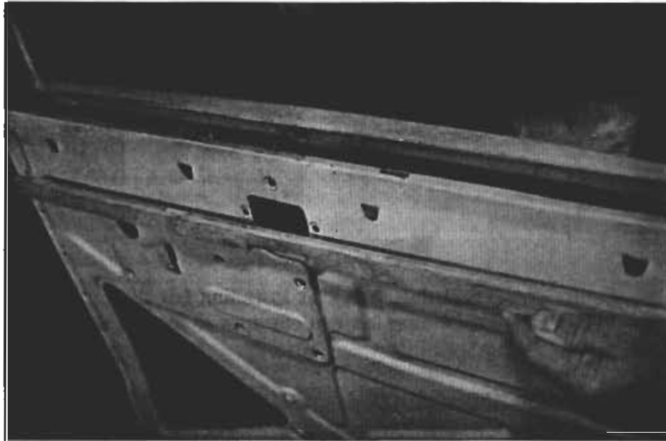
Figure (8) Wooden tack strip to be installed in inner top edge of door
