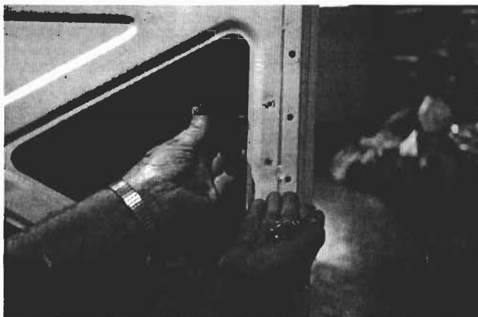
Figure (20) Rear down-stop bracket installation
